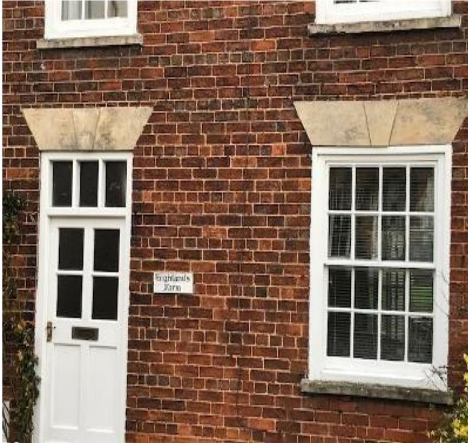
Traditional door, wooden window frame and stone lintel
