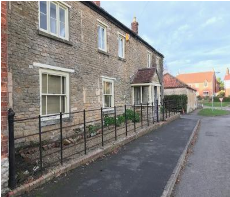
Local stone and traditional plain lintels
