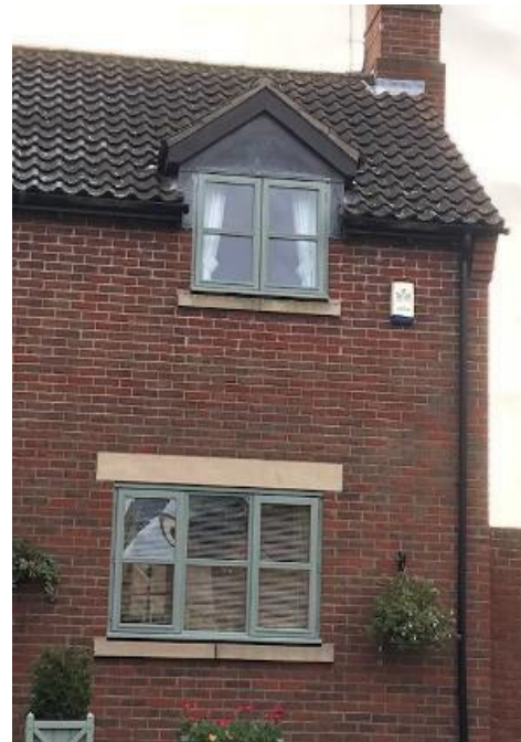
Modern dormer copy, modern brick and modern lintel
